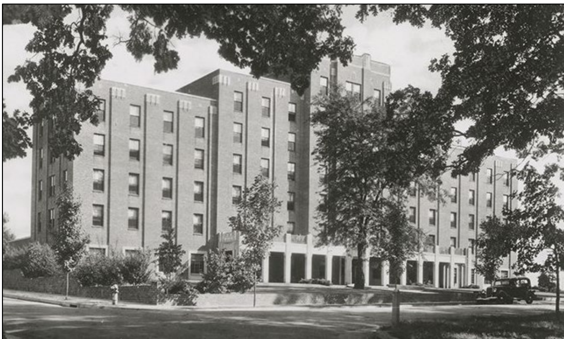
Figure 4: 1930s photograph of The Virginia Home for Incurables. Source: The Virginia Home Archives
