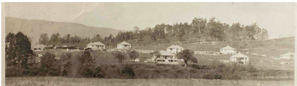
Figure 7 – Bacova employee housing under construction in 1920 looking roughly north from the current location of Lake Bacova. Lumber is stacked on the left side of the image waiting to be assembled. Courtesy Bath County Historical Society.
