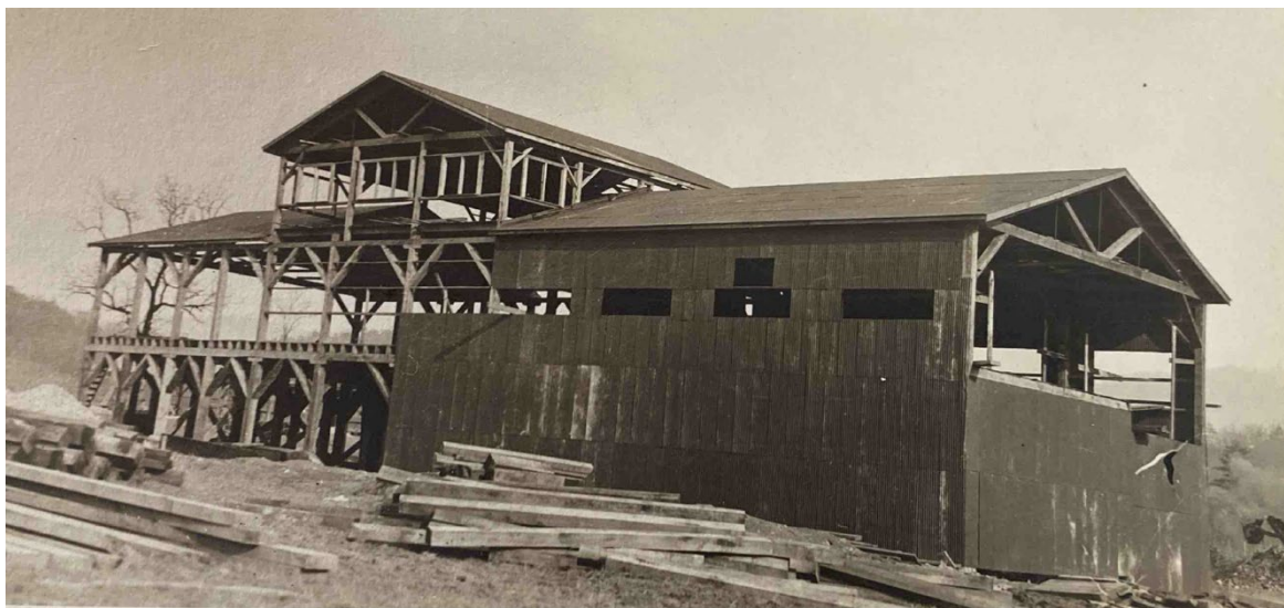
Figure 6 – First mill building under construction in 1920-1921. This two-story building was located immediately south of the existing brick power plant building. Courtesy Bath County Historical Society.
