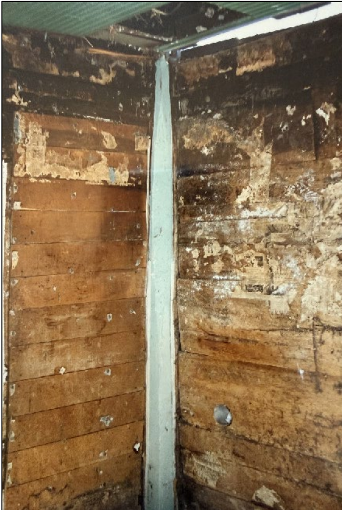
Figure 2. Plank north wall (right) of kitchen before being dismantled ca. 1991.
