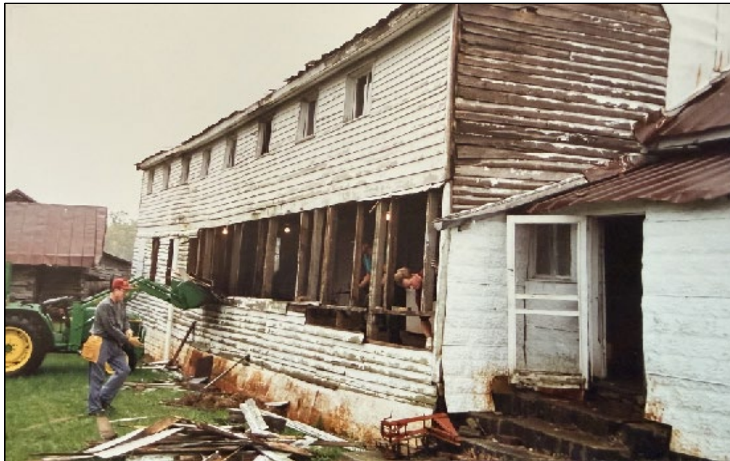
Figure 3. Rear porch being dismantled, circa 1991.
