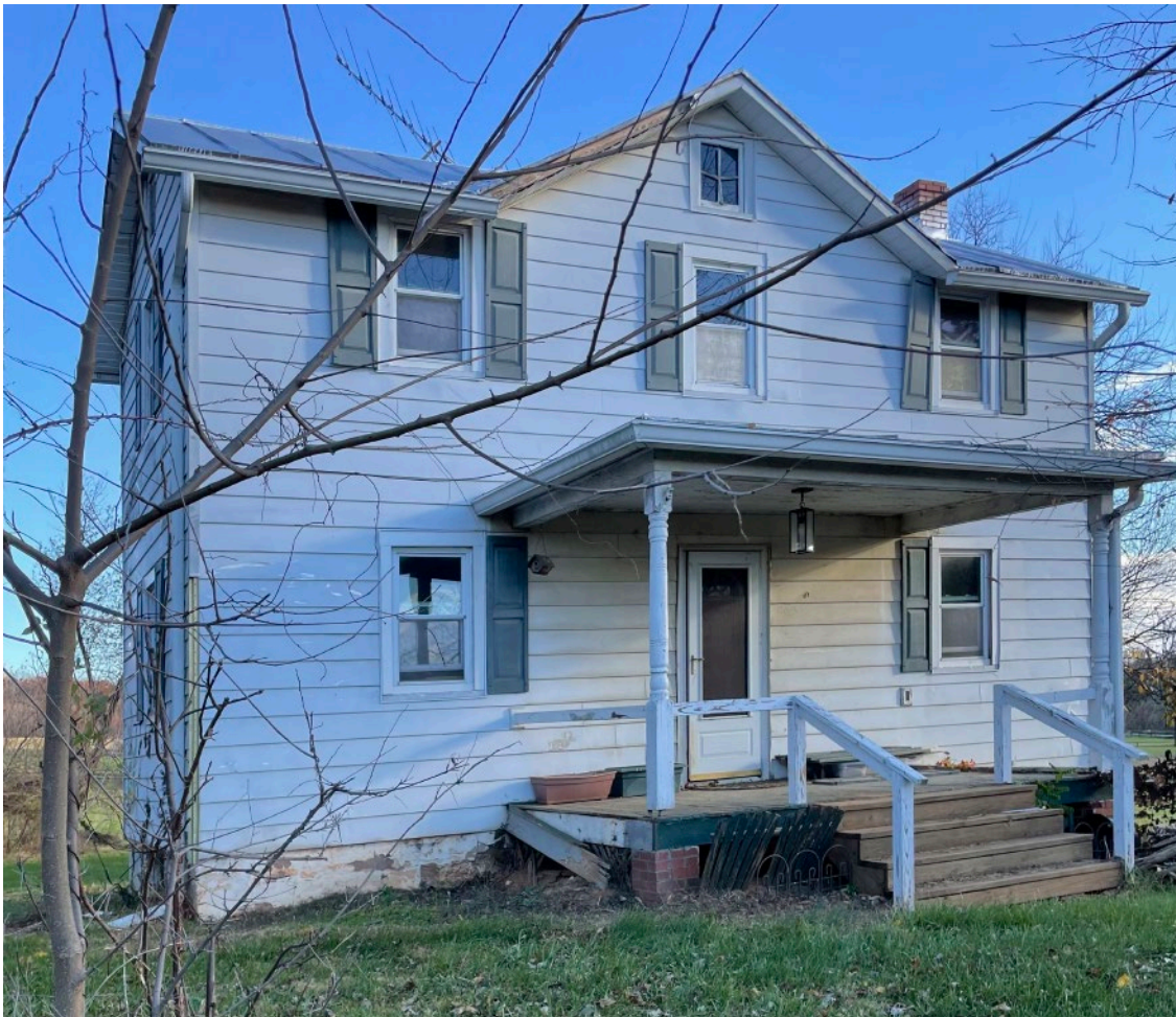
EXHIBIT 15B: TENANT HOUSE (PRESENT DAY)
