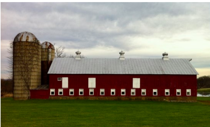
EXHIBIT 10: DAIRY BARN WEST FACADE
