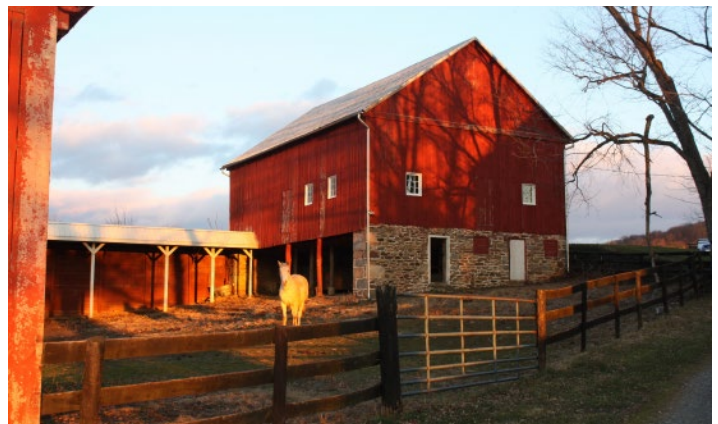
EXHIBIT 11: BANK BARN LOOKING N-W
