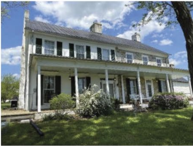
EXHIBIT 45: BALLROOM / MAIN HOUSE
