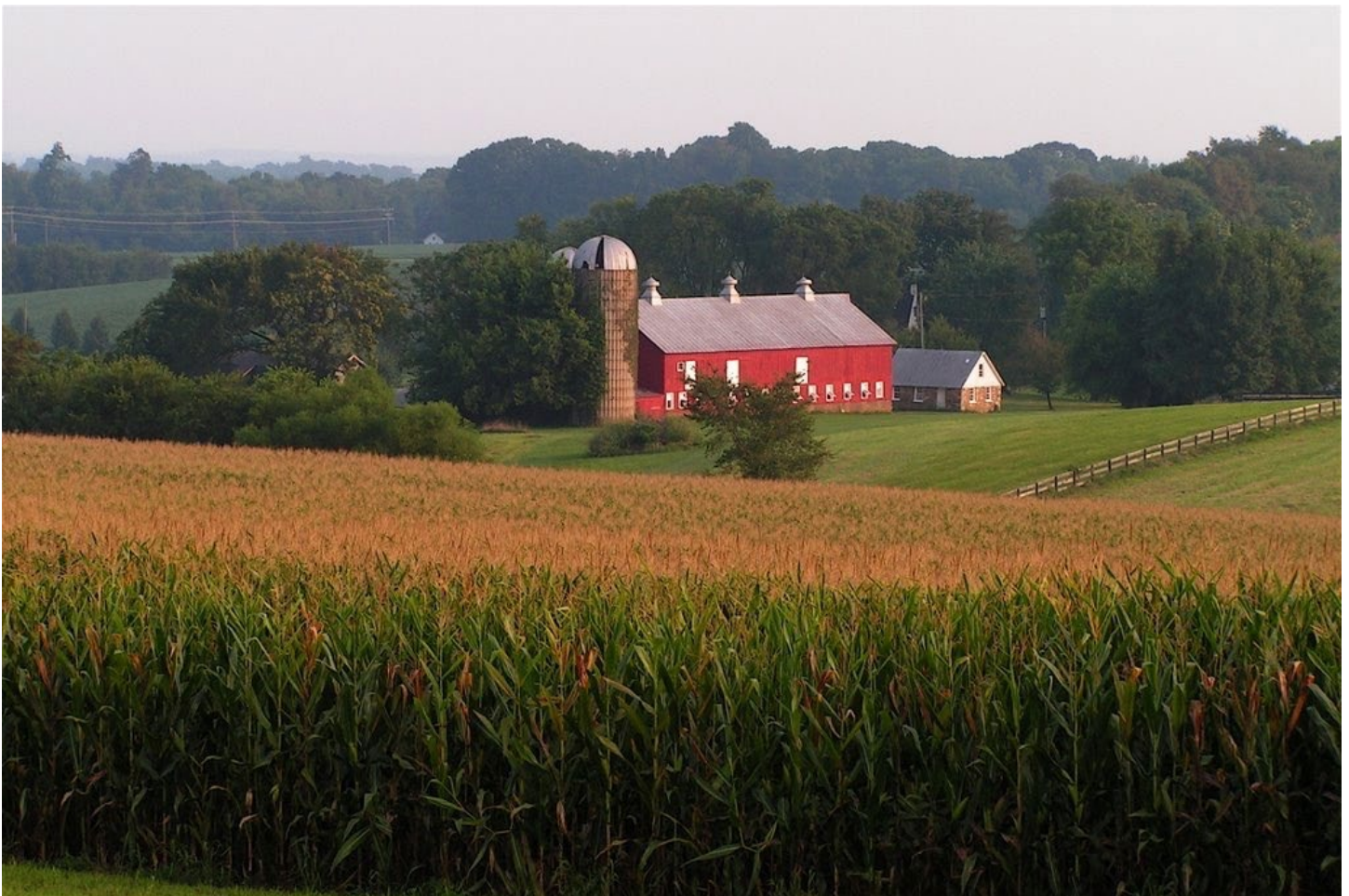
EXHIBIT 17: VIEW OF DAIRY BARN AND MILK HOUSE LOOKING SOUTH-EAST
