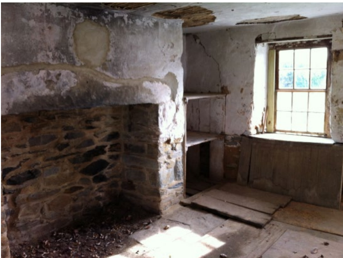
EXHIBIT 43: STONE KITCHEN LOOKING S-W
