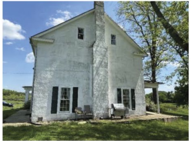
EXHIBIT 46: BALLROOM WEST FACADE
