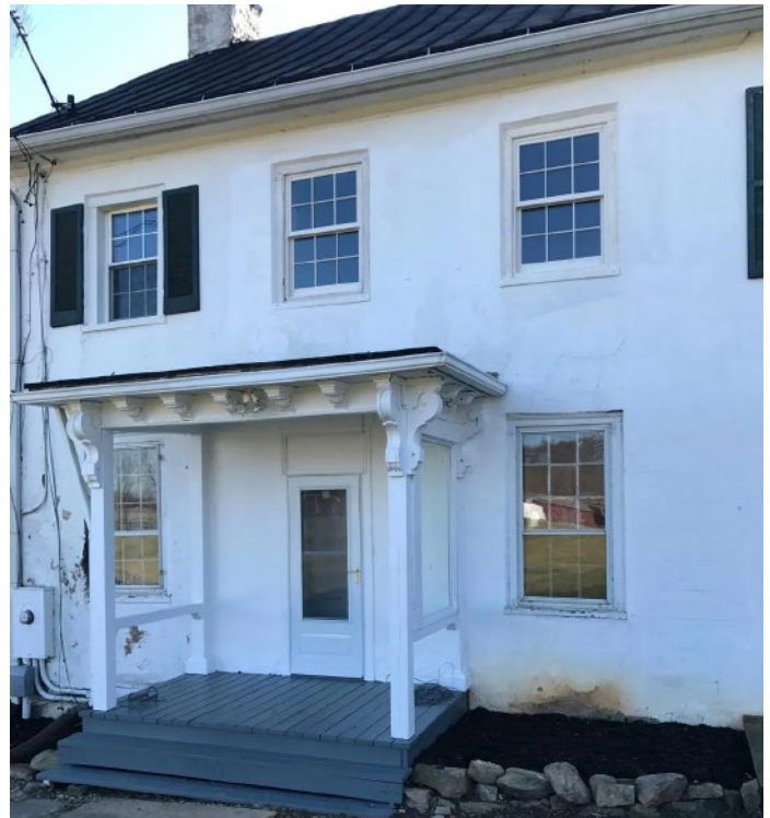
EXHIBIT 7: MAIN HOUSE NORTH DETAIL
