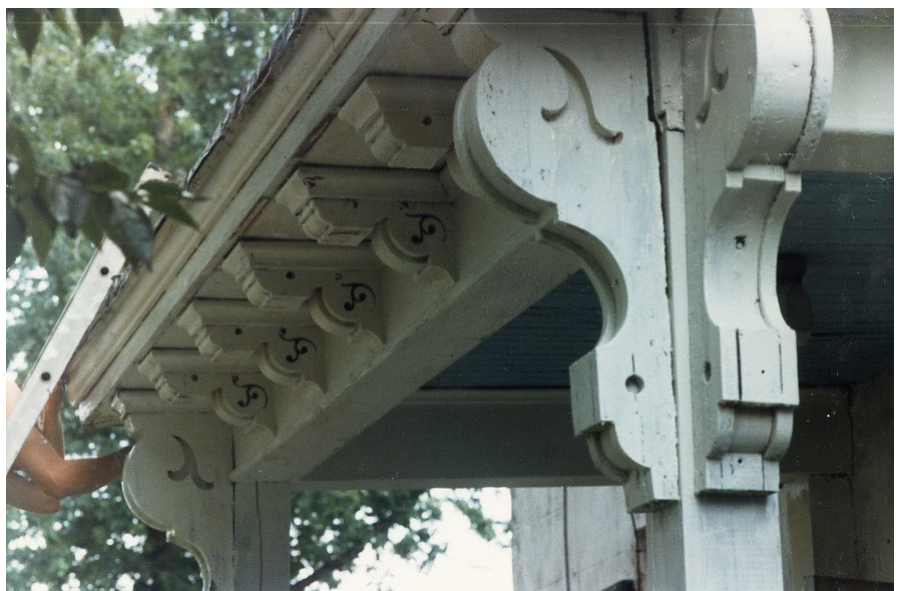
EXHIBIT 32: REAR PORCH DETAIL
