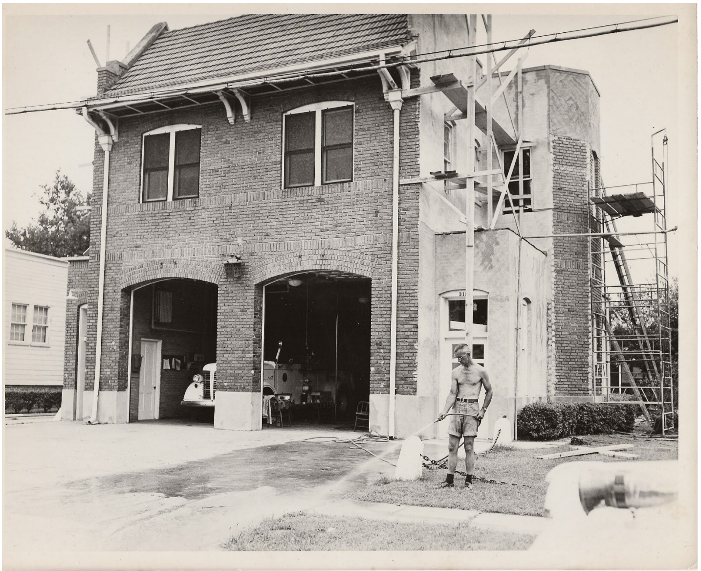
Figure 2: Fire Station No. 11 in ca.1959 taken while stucco finish was being applied to the exterior. Courtesy of Norfolk Fire Department.
