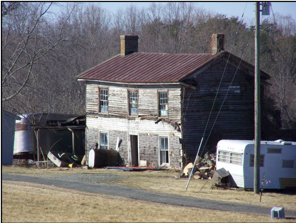
Figure 25. Rocky Pin (VDHR #089-0272), Sanford Drive, View Looking Southwest.
