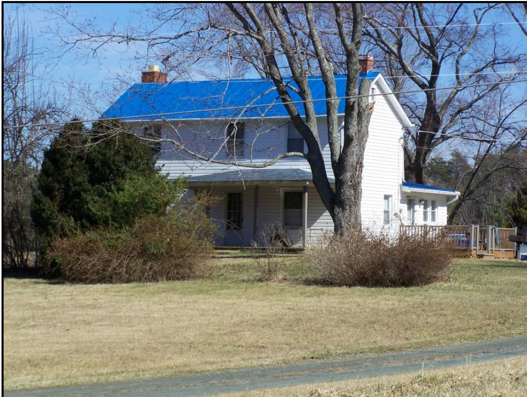
Figure 15. Farm (VDHR #089-0192), 2582 Mountain View Road, View Looking East.
