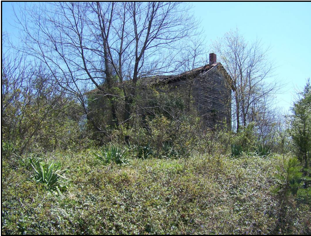
Figure 31. Farm (VDHR #089-5393), Mountain View Road, View Looking Southwest.
