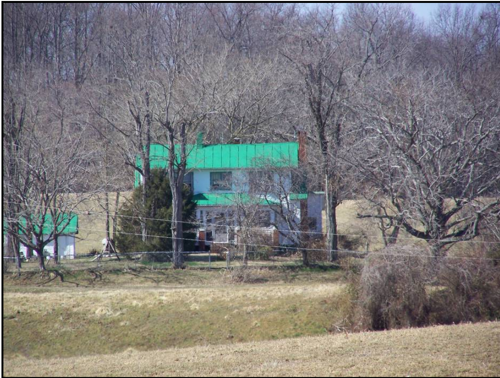
Figure 23. Poplar Grove (VDHR #089-0218), 1499 Poplar Road, View Looking Southwest.
