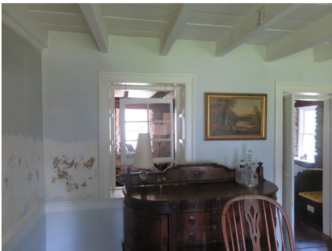
Figure 1. Photo taken of preserved window opening of the first addition, now looking into the sitting room of the second addition. 8
