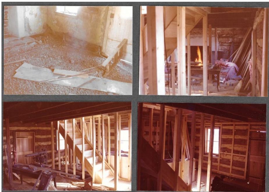
Figure 3. Images taken by William Miner of remodeling the house's first and second floors and installing the new staircase. 12
