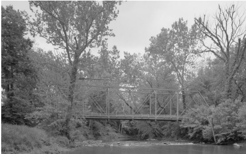
A 1968 photo of the iron truss bridge over Catoctin Creek near Waterford
