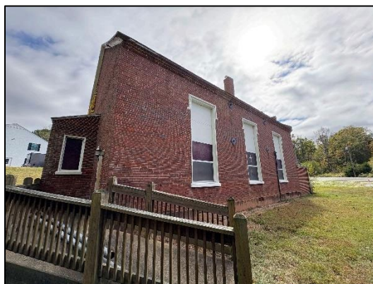
Figure 3: West elevation, facing southeast.
