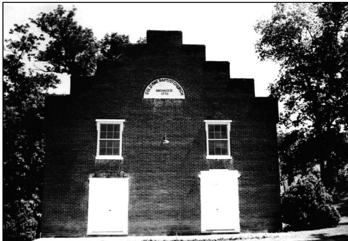
Figure 2: Façade prior to the addition of the vestibule, photographed in 1968 by K. Read, facing north.
