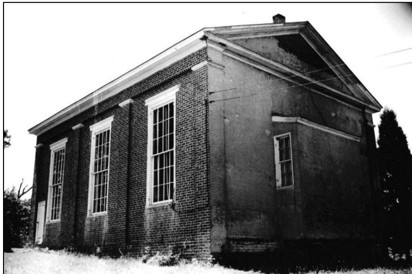
Figure 12. East and north elevations of Lasley Meeting House, photographed in 1968 by K. Read.
