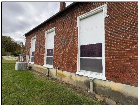
Figure 4: East elevation, facing southwest.
