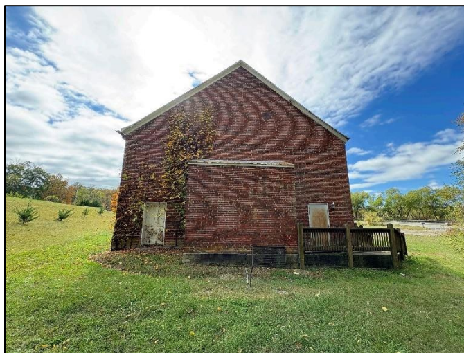
Figure 5: Rear elevation, facing south.
