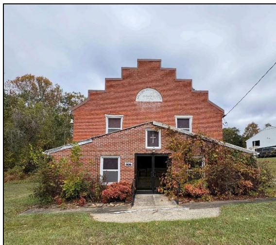
Figure 1. Façade featuring the vestibule added in the 1970s, facing north.
