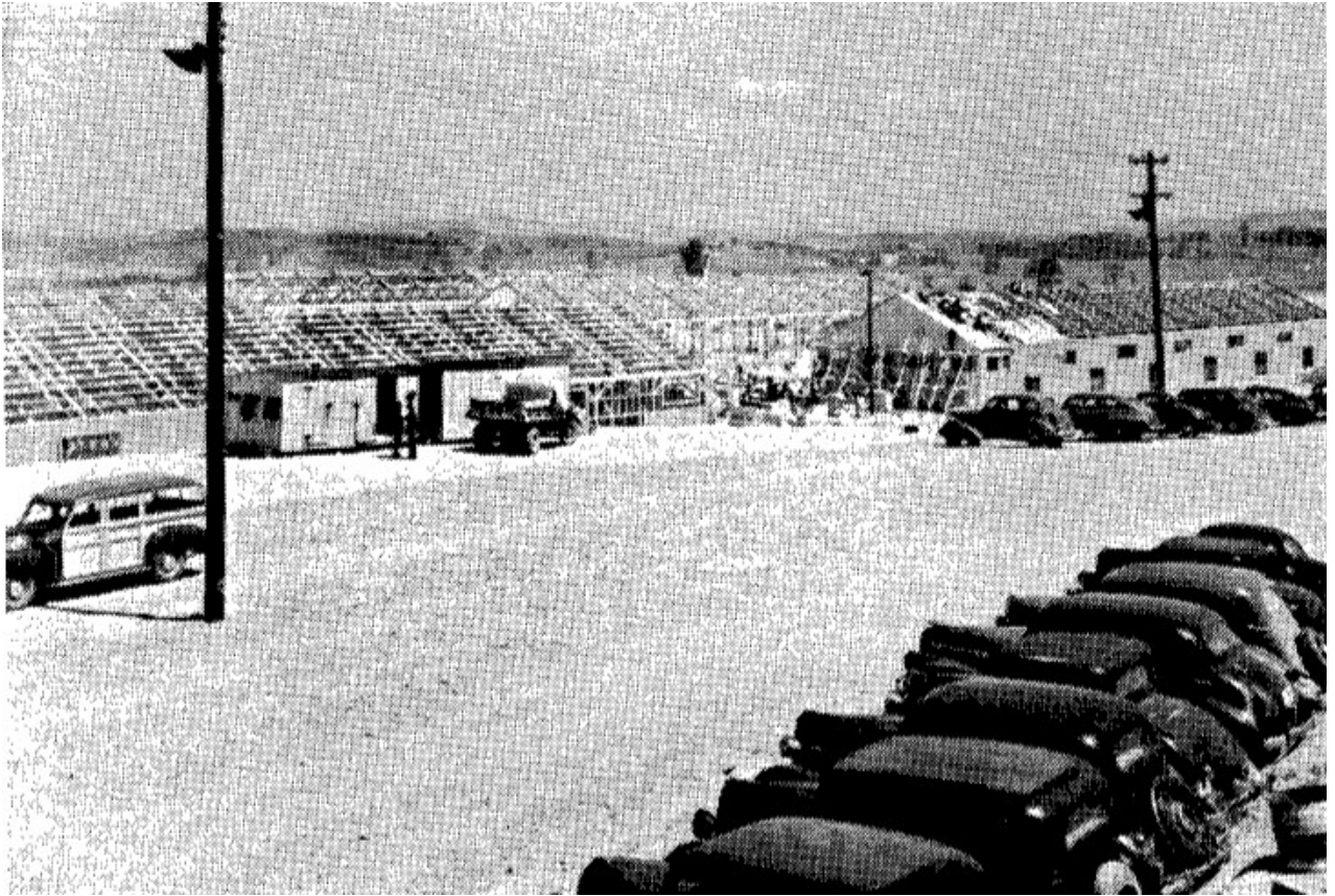
Figure 2: NROP Construction May 15, 1941
