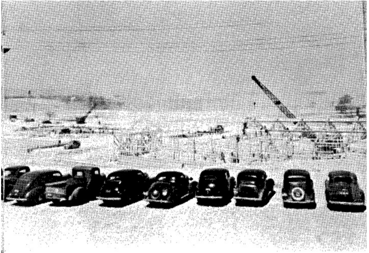
Figure 1: NROP Construction May 15, 1941
