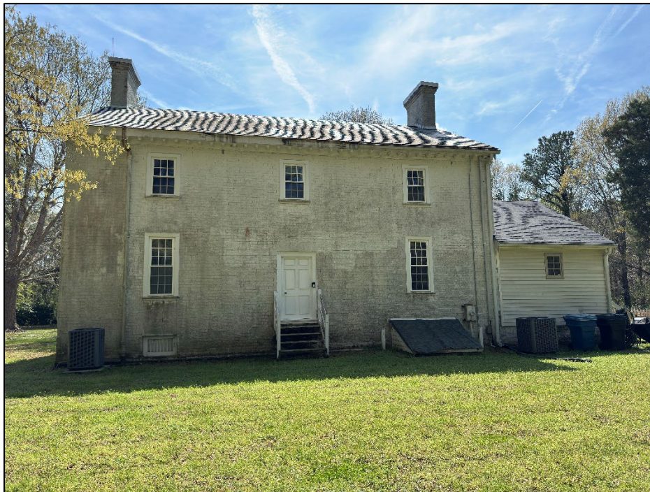
Upper Wolfsnare, north elevation, March 2026. Photo by the author.
