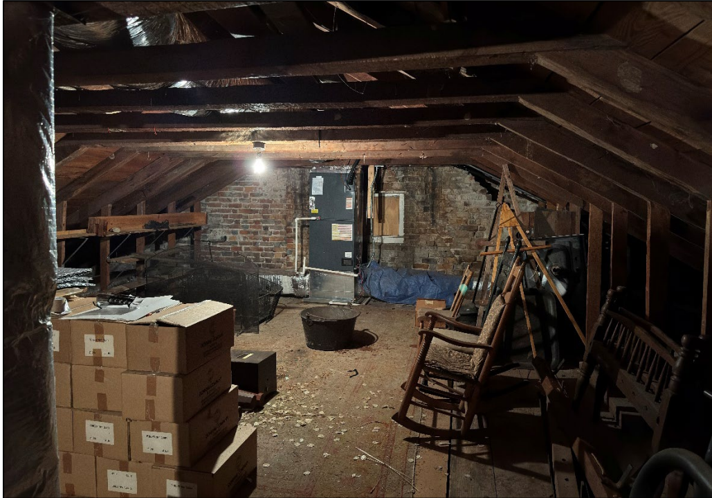
Upper Wolfsnare, attic, looking at the west end wall, November 2025. Photo by the author.
