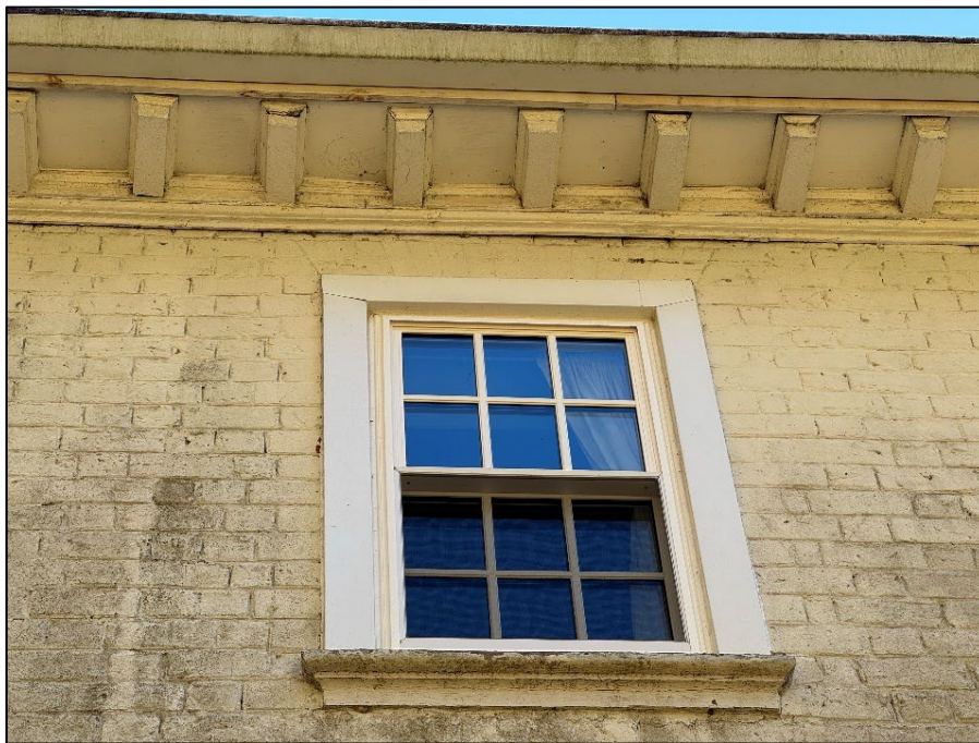
Upper Wolfsnare, North elevation window and cornice detail, November 2025. Photo by the author.
