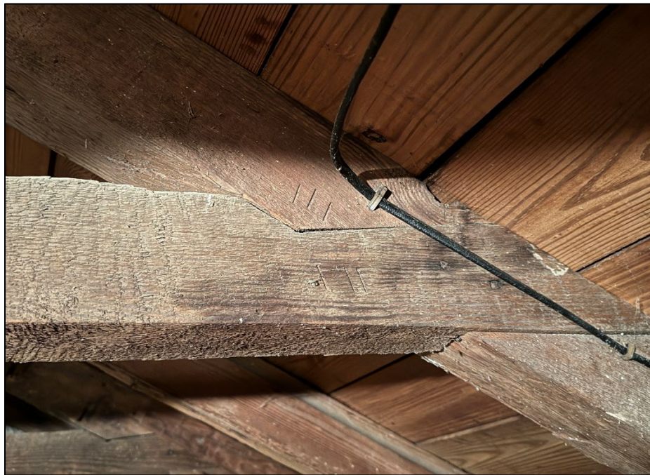
Upper Wolfsnare, roof framing as seen in the attic, carpenter's mark indicating matching collar tie and rafter, November 2025. Photo by the author.
