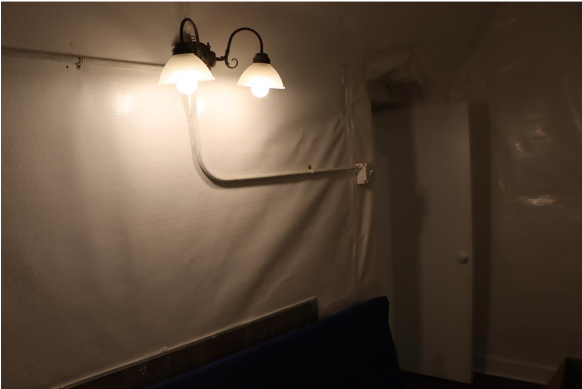
Carriage House, basement, enclosed horse alley, south wall, 5/16/2026
