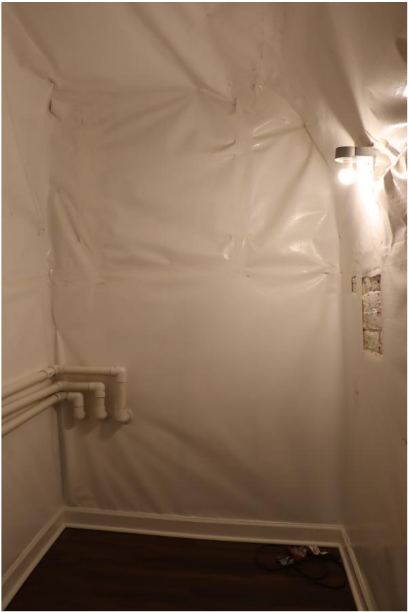
Carriage House, basement, enclosed horse alley, 5/16/2026
