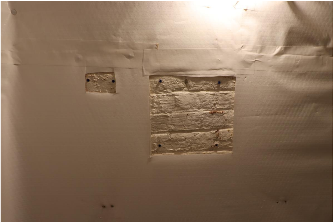
Carriage House, basement, enclosed horse alley, north wall, 5/16/2026
