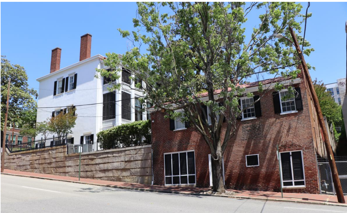
Barret House and Carriage House, south elevation, 5/16/2026
