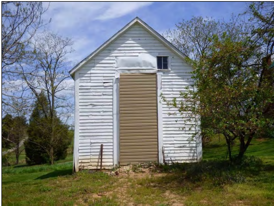
Photo 83: Location of Demolished Chimney, West Elevation.
