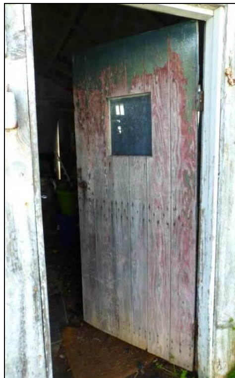
Photo 64: Door Detail on West Elevation of Kitchen.
