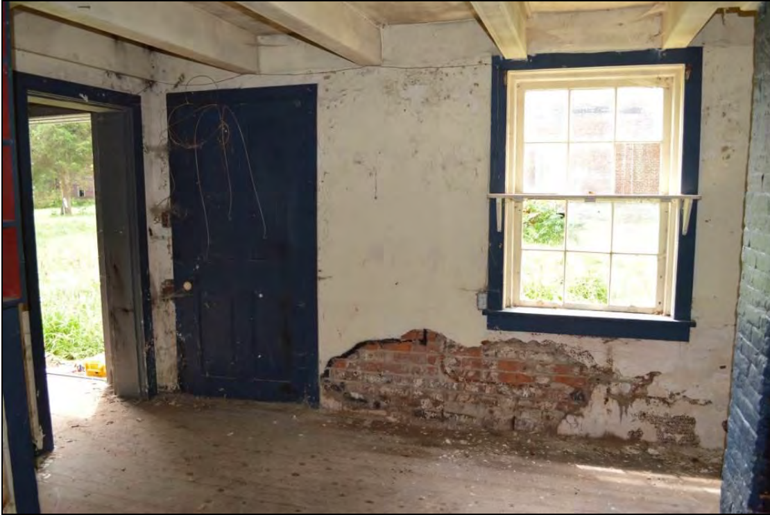
Photo 39: South Wall in West Room of Kitchen/Quarter.
