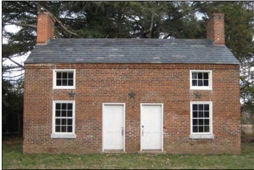
Photo 35: Sherwood Forest Kitchen/Quarter, Primary (South) Elevation.
