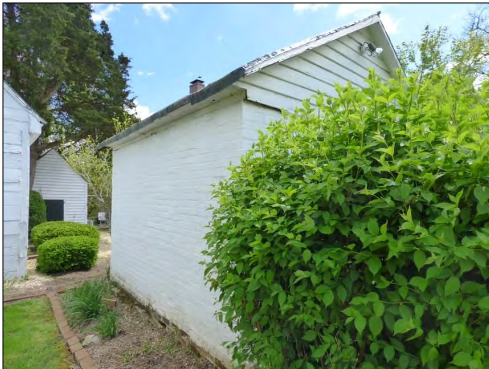
Photo 20: Carlton Dairy, North Oblique.
