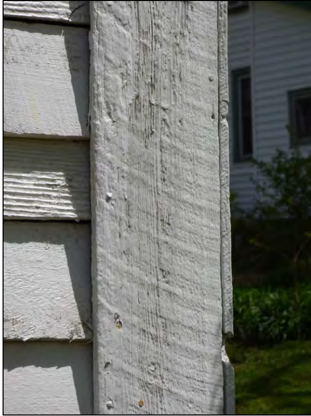
Photo 82: Circular Saw Mark Details on Northeast Elevation.
