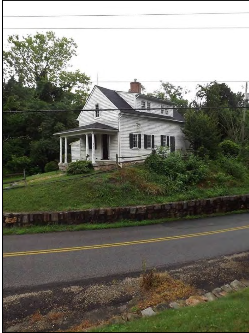
Photo 40: Caretakers Cottage, Southwest Oblique.
