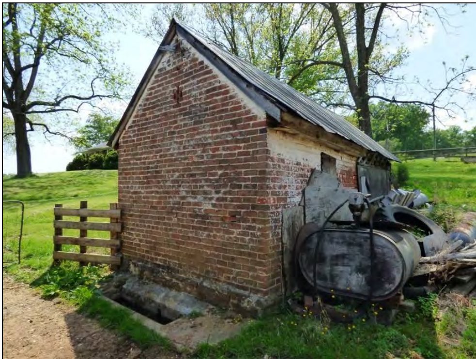
Photo 75: Spring House, Northwest Oblique.
