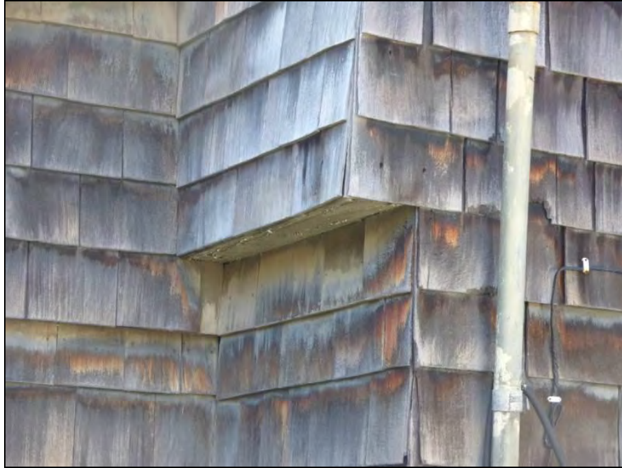
Photo 45: Jettied Construction Detail on Northeast Elevation.
