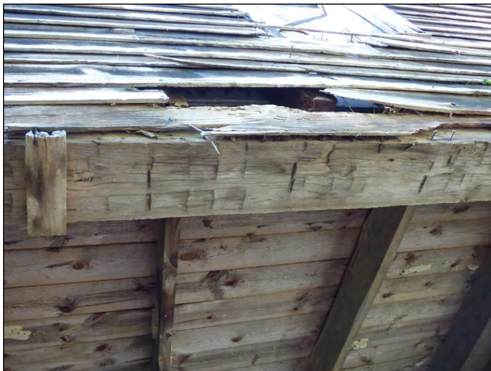
Photo 110: Saw and Adze Marks on Southwest Elevation.
