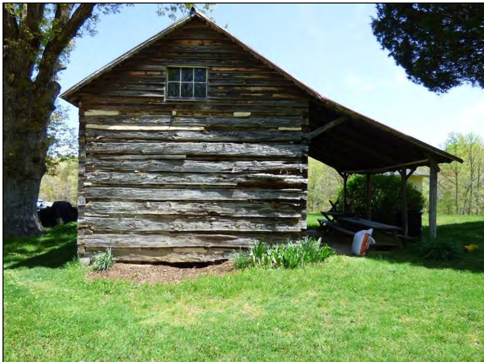
Photo 92: Patton Outbuilding, South Elevation Shed Roof.
