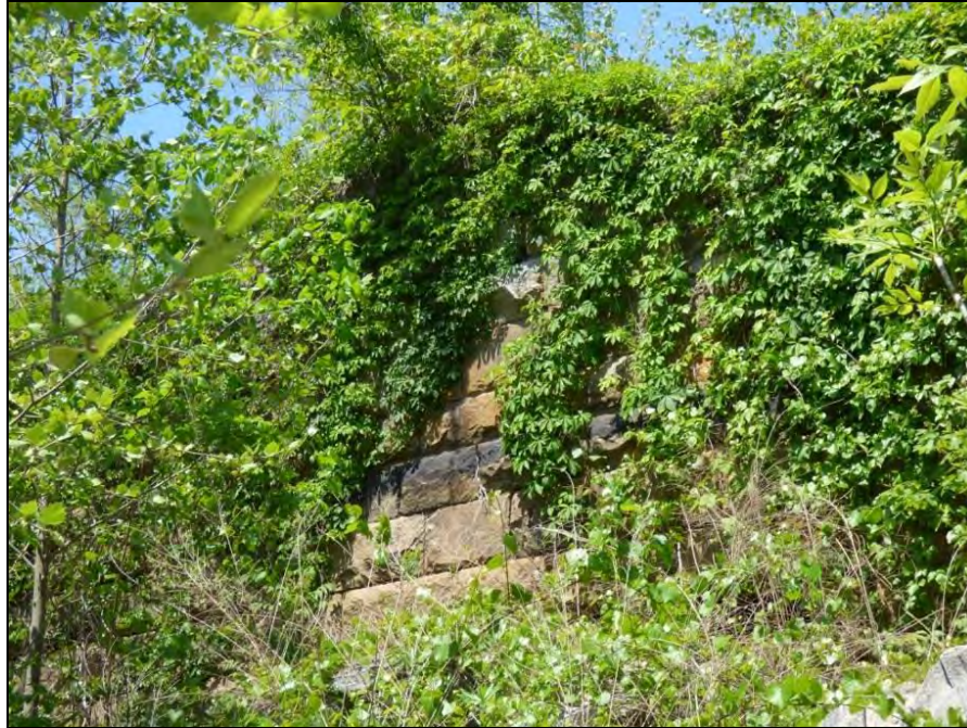
Photo 73: Hunters Dam Stone Wall, Looking Northwest.
