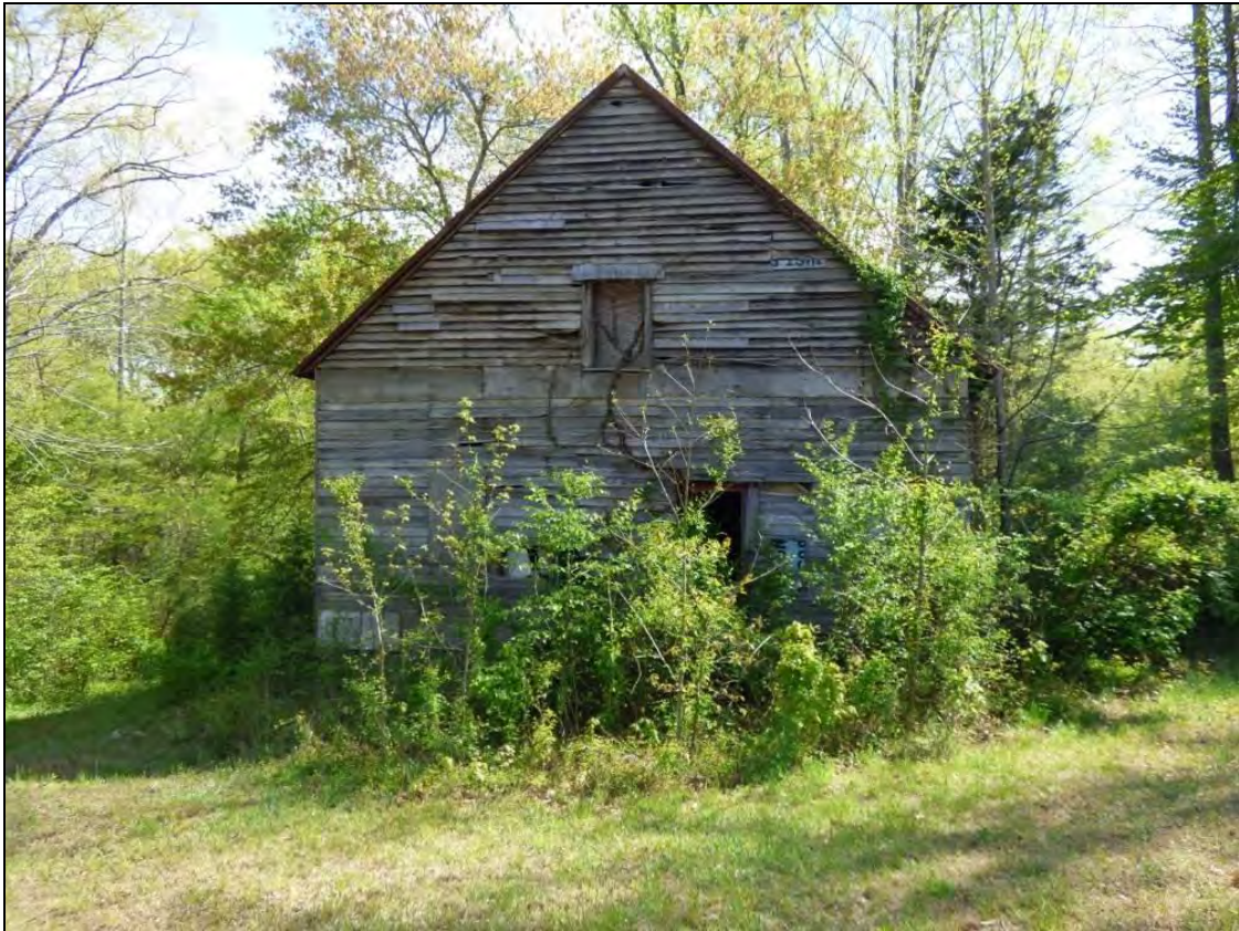
Photo 108: Kendall's Mill, Northeast Elevation.
