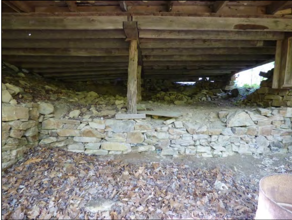
Photo 109: Structural System, Looking Northeast.
