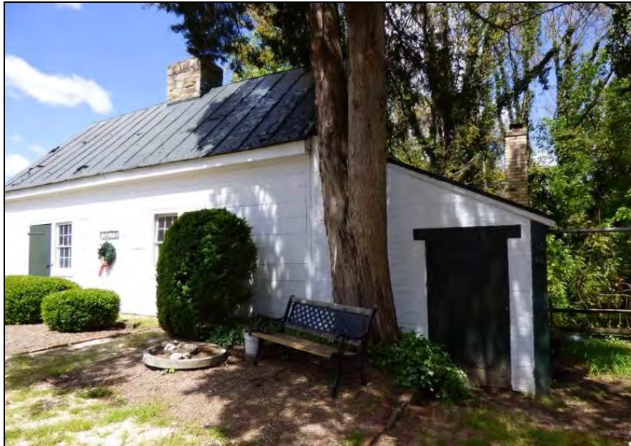
Photo 14: Kitchen/Quarter Addition, Looking North.
