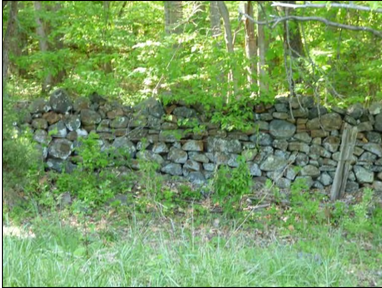
Photo 80: Detail of the Stone Wall, Looking Northwest.
