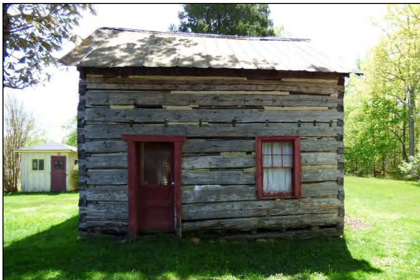
Photo 88: Northeast Elevation of the Patton Outbuilding.
