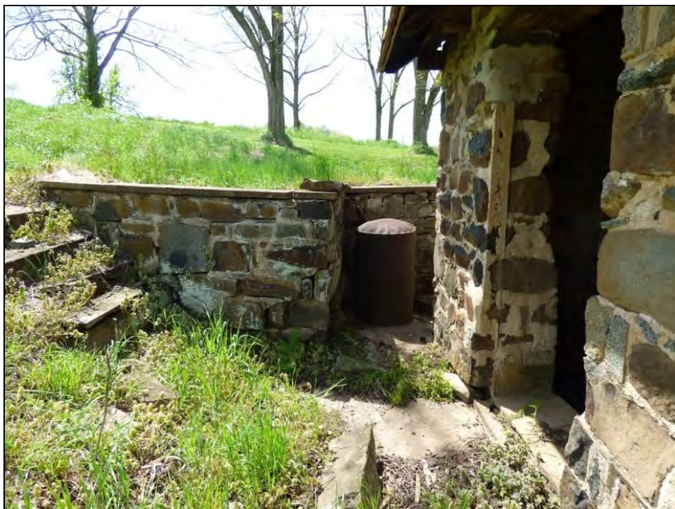
Photo 86: Retaining Wall, Looking West.
