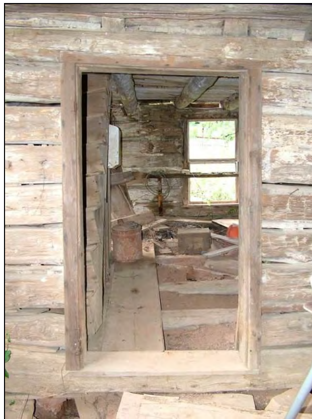
Photo 96: North Doorway Detail.
