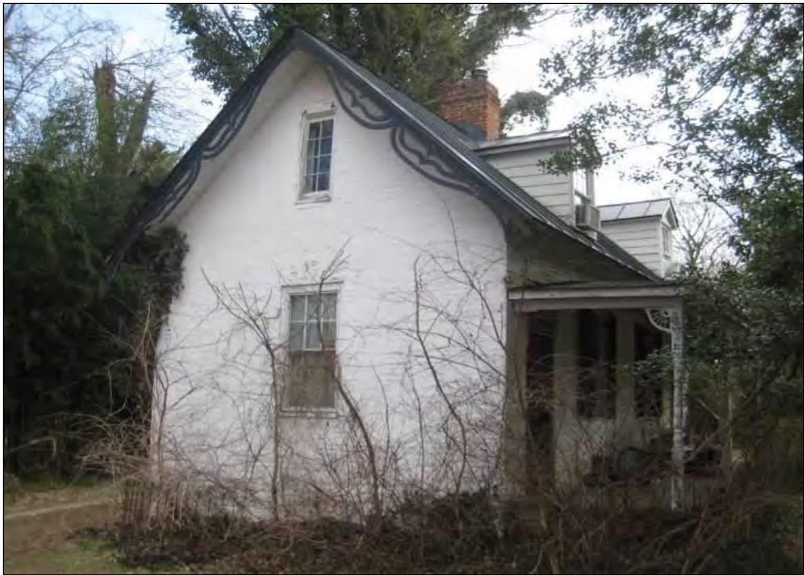
Photo 25: Phillips House Slave Duplex, West Elevation.
