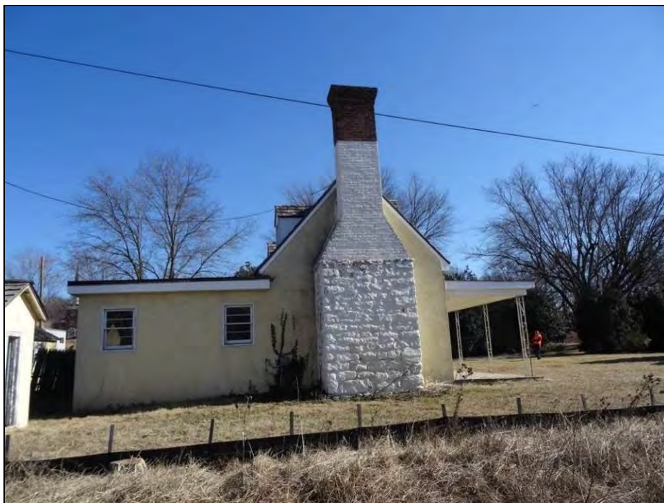
Photo 51: Dunbar Kitchen/Quarter, Northwest Elevation.
