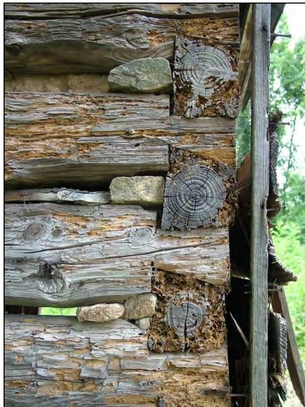
Photo 98: Dovetail Notching Detail.
