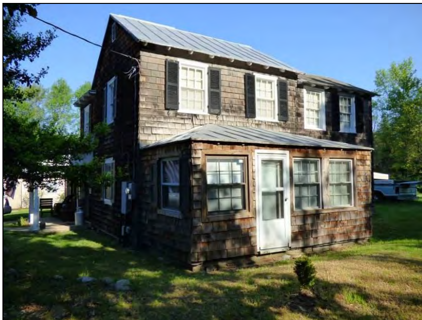
Photo 47: Additions on 50 Caisson Road, Southeast Oblique.
