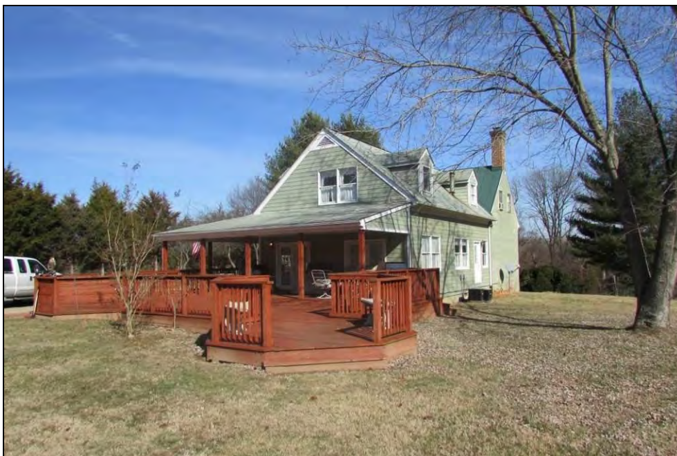
Photo 62: Addition and Deck, South Oblique.
