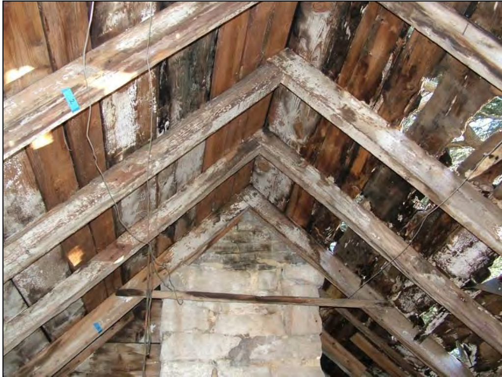
Photo 33: Roof Frame of the Duplex.
