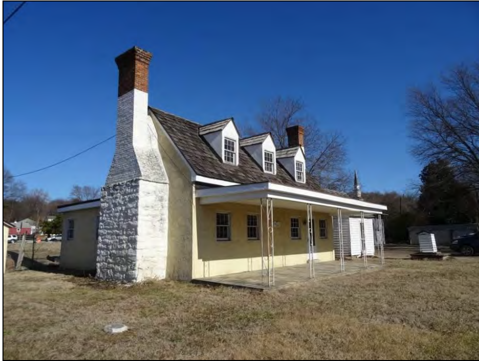
Photo 50: Dunbar Kitchen/Quarter, West Oblique.
