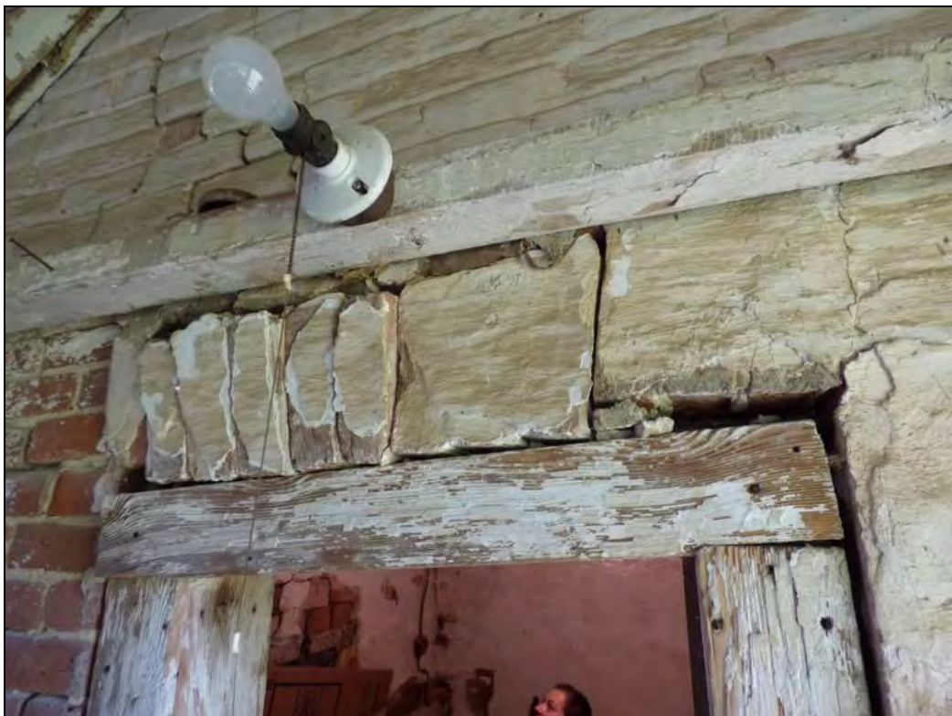
Photo 77: Spring House, Jack Arch Detail on Interior.
