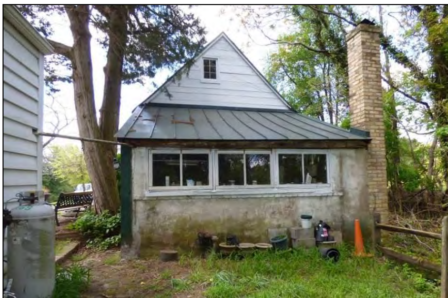
Photo 15: Kitchen/Quarter Addition, Southeast Elevation.
