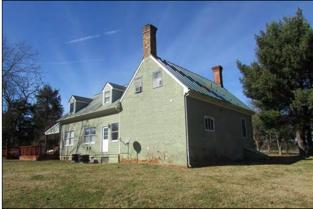
Photo 59: Hollywood Kitchen, East Oblique.
