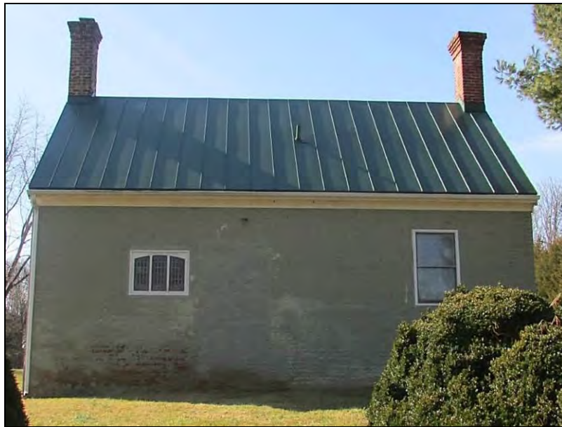
Photo 56: Hollywood Kitchen, Northeast Elevation.
