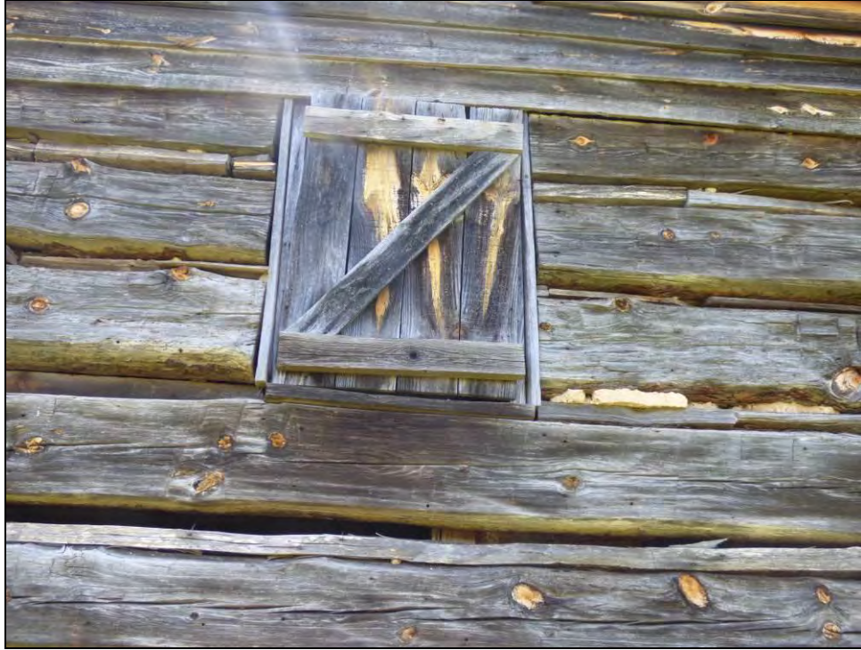
Photo 91: East Elevation Detail.
