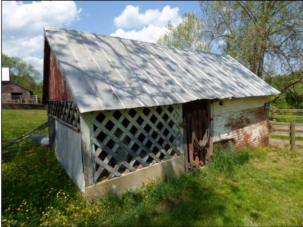
Photo 74: Walnut Hill Spring House, Southwest Oblique.
