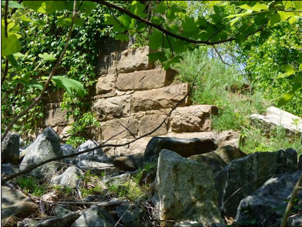
Photo 71: Hunters Dam Stone Wall, Looking Northwest.
