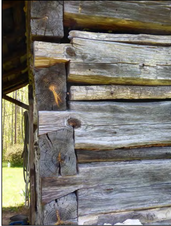
Photo 89: Half-Dovetail Notching at the Corners of the Building.
