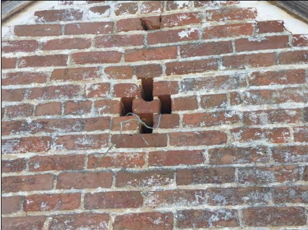
Photo 76: Spring House, Brick Detail on East Elevation.
