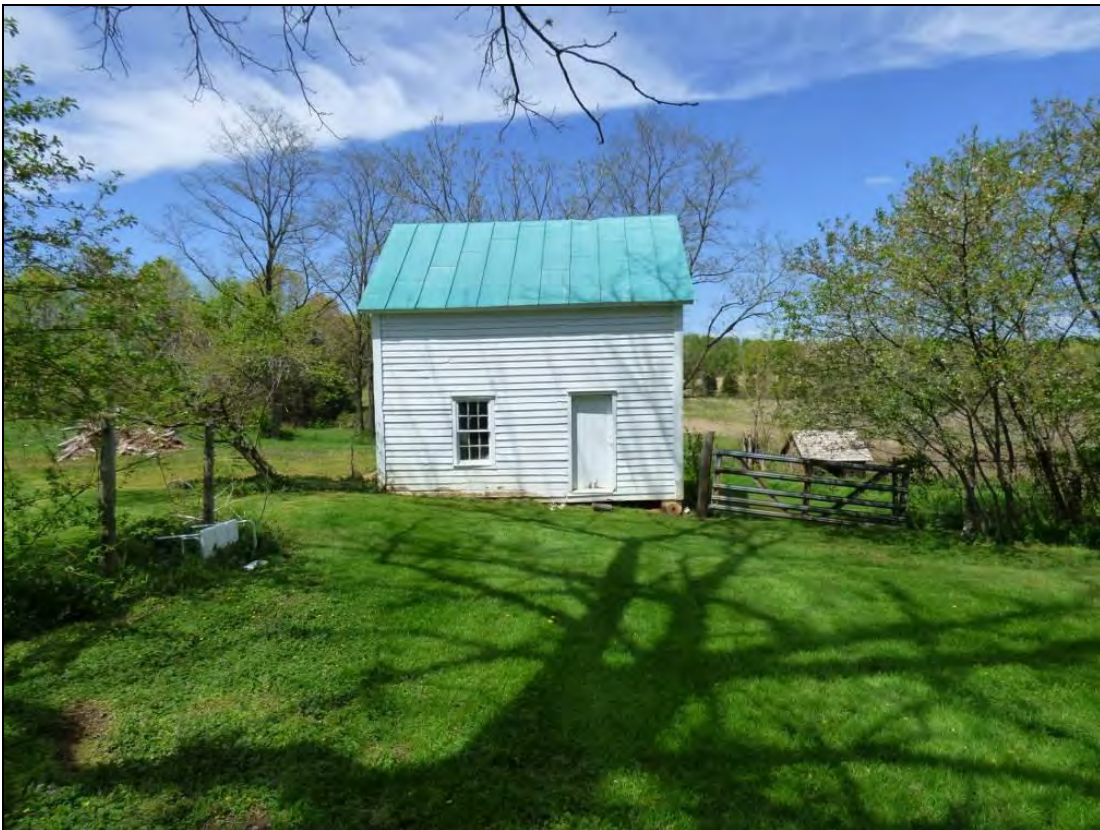
Photo 81: Poplar Grove Kitchen/Quarter, Primary (Southeast) Elevation.
