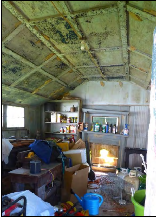
Photo 67: Interior of Kitchen, Looking East.
