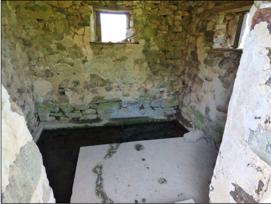
Photo 87: Interior Detail, Looking North.
